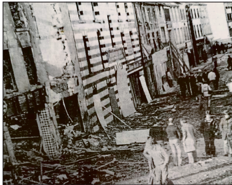
A scene which was all too familiar in the 1980s. In this case the Ulster Gazette's offices in Scotch Street were badly damaged following a bomb. Despite these attacks the Ulster Gazette always made it onto the shop shelves.
